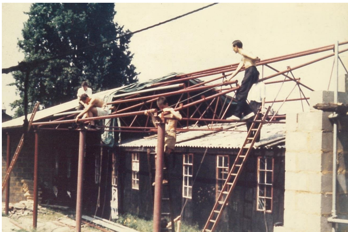
Figure 14 – Building the new HQ over the top of the old building (1965) including Geoff Collins (far right) and Les Kingswood (second from right)
