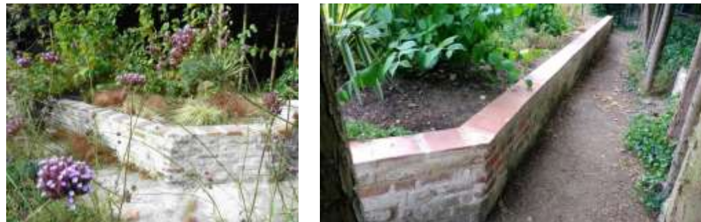
After – completed in June 2017
