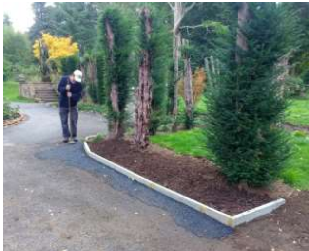
October – New edging installed by Yew Room.
