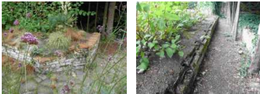
October – Low Greenhouse Wall renovation – Before
