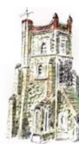
17 Old Church Tower
