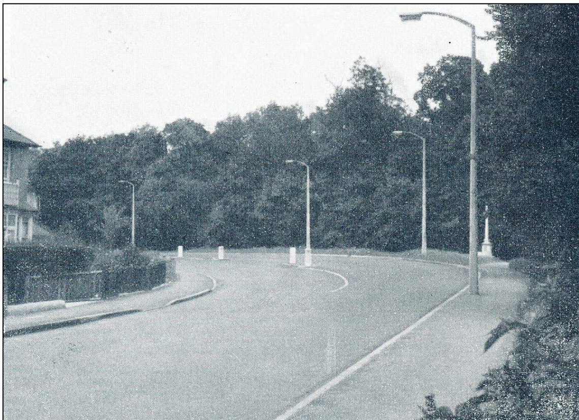
London Road, Ewell – A recent road improvement
