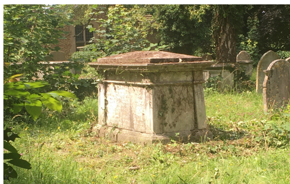
. . . and in July 2021, done and dusted.
