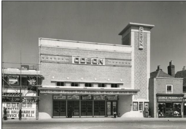
The Odeon, Epsom High Street (Demolished in 1972)
